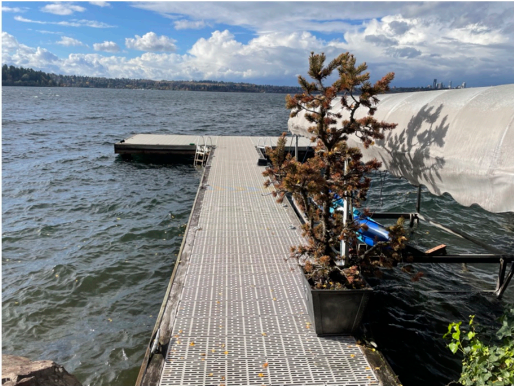
Photo 1 - Pier looking water ward.
